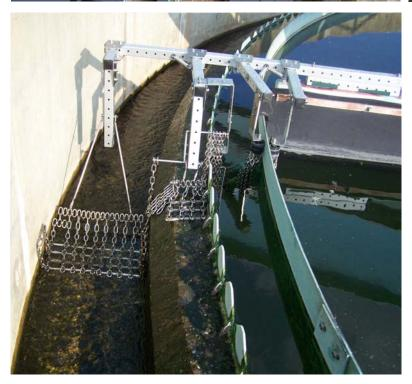
Clarifier CleanSweep<sup>TM</sup> The new consists of a tubular aluminum frame which cleaning from the various elements function. Components consist of horizontal and vertical sweeping chains for troughs spillways, and a unique rotating chain device to clean the trough walls, weir plate, and both sides of the baffle ring. All components are constructed of aluminum and stainless steel, with surfaces fabricated from wetted stainless steel.
