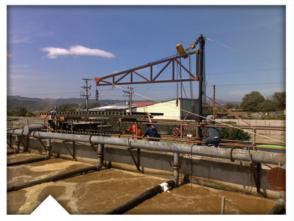
Retrievable grid with SSI Snappy Saddle™ Diffusers and a 304 SS frame replacing an underperforming floating lateral system
