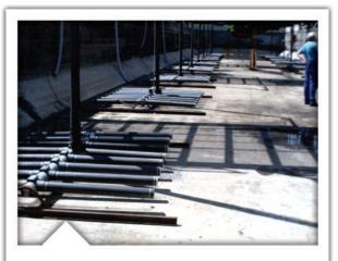
These liftable fine bubble tube grids on guide rails have worked over 10 years in this municipal WWTP
