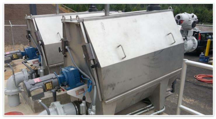
The highly efficient Internally Fed Drum Screen offers low water usage and low energy consumption, while maximizing screening efficiency.
