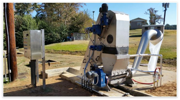
The Kusters Water ProTechtor<sup>™</sup> Screenings Washer Compactor is known for its reliable operation and robust design. The washer compactor significantly reduces screenings volume while simultaneously removing organic content, resulting in cleaned and dried screenings. All ProTechtor<sup>™</sup> products are US Manufactured at Kusters Water's ISO 9001:2008 certified facility.
