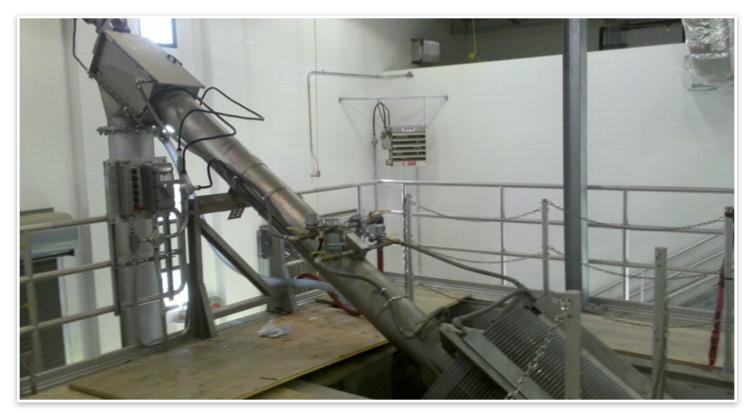
The In Channel Drum Screen is suitable for treating flow rates up to 45 mgd per screen.
